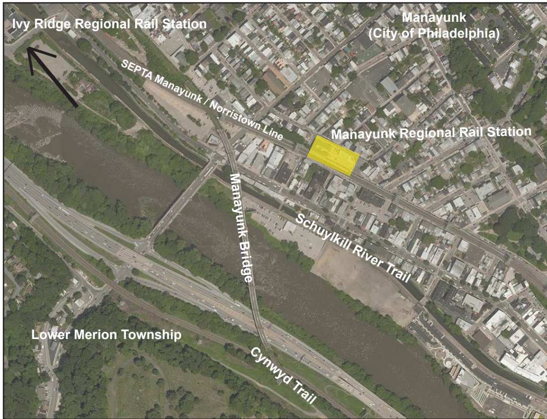
FIGURE 5: AERIAL OF MANAYUNK BRIDGE TRAIL NETWORK
