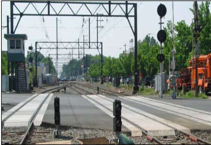
R5 Main Street (Lansdale) Grade Crossing Improvements
