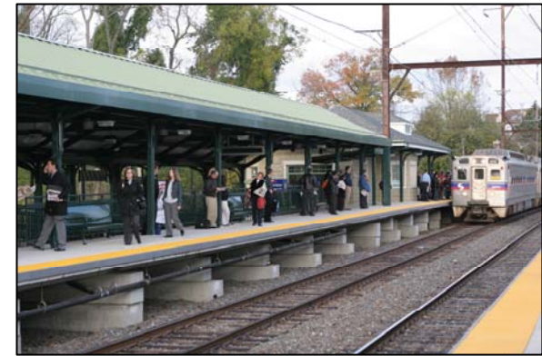
R5 Fort Washington Station
