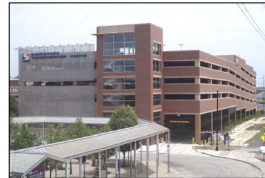
Norristown Transportation Center Parking Garage
