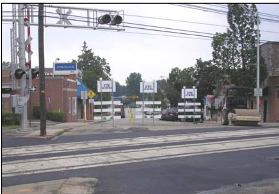
Route 101 Media Line Saxer Avenue Grade Crossing Renewal
