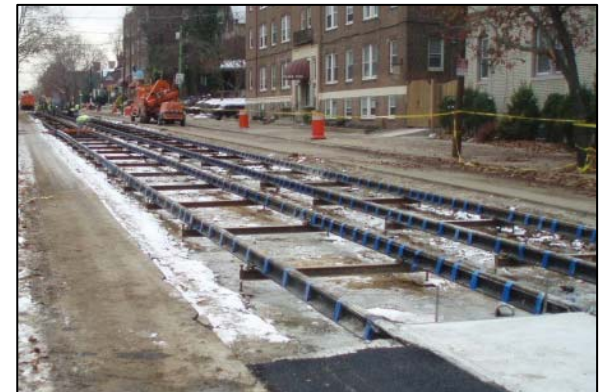
Route 13 Chester Avenue Track Renewal
