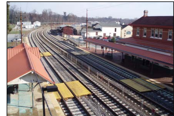
R5 Paoli Line Continuous Welded Rail and Concrete Cross-ties
