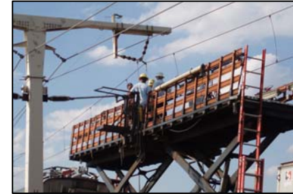
R1 Airport Line Catenary Replacement
