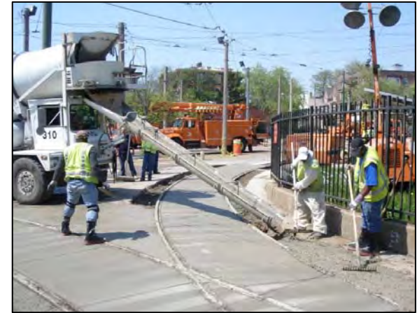
Special Trackwork Renewal 40th Street Trolley Portal
