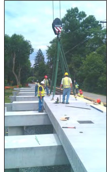
Ryers Station Reconstruction
