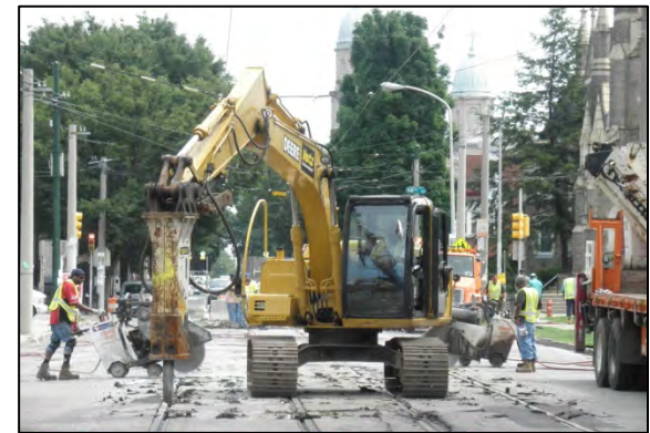
58 th and Chester Avenue Track Renewal Project
