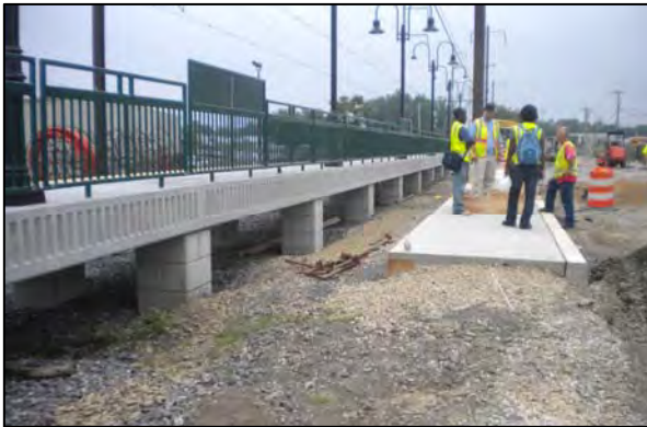
Primos Station Reconstruction
