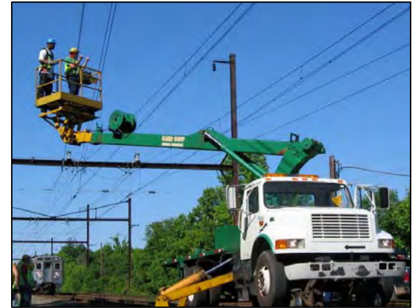
Catenary Replacement Doylestown Line
