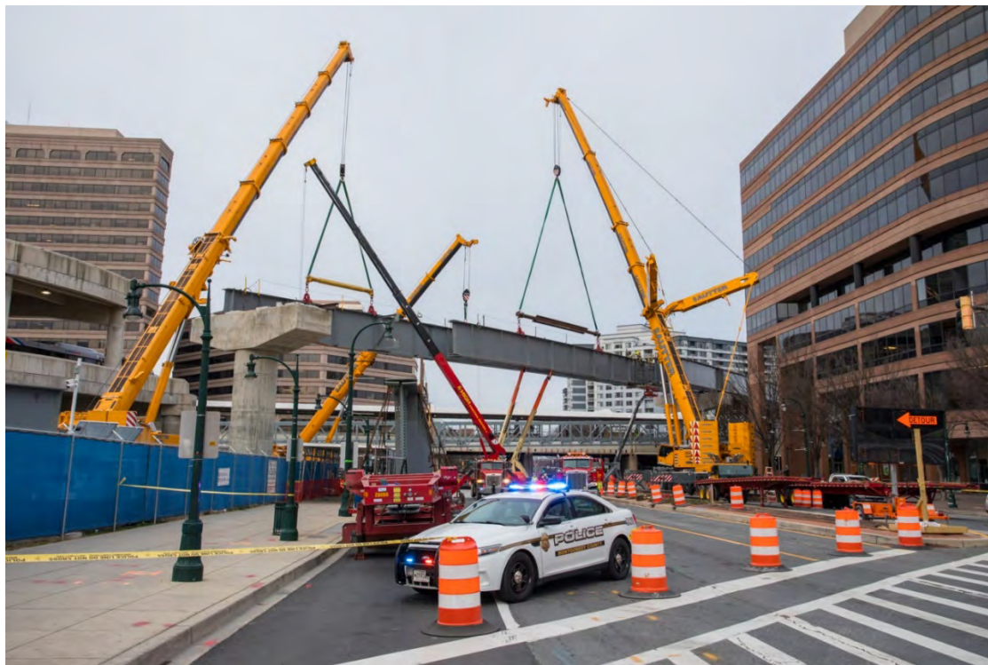
Figure 2.3-19: Elevated Guideway Construction
