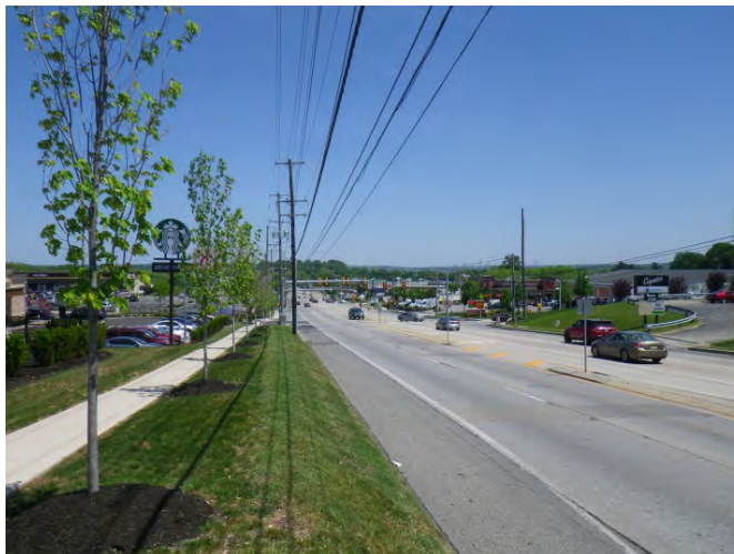
Figure 4.8-6: VAU 6 – US Route 202
