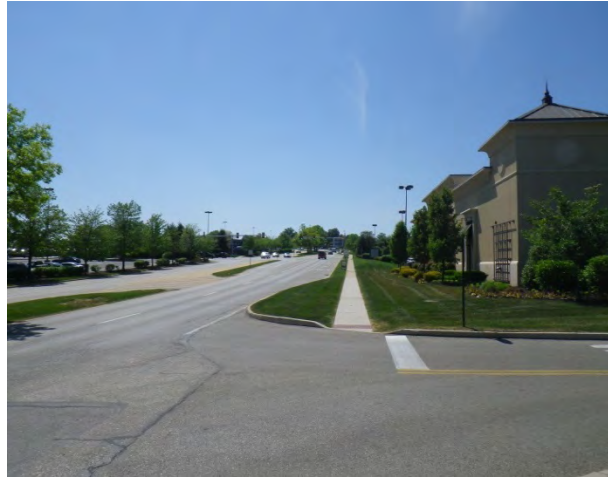
Figure 4.8-2: VAU 2 – King of Prussia Mall Area
