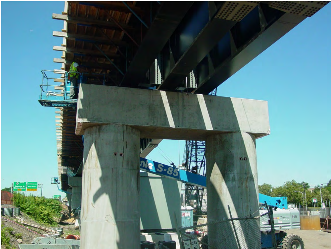
Figure 2.3-20: Elevated Guideway Construction
