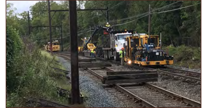
Doylestown & Warminster Tie Renewal (Complete)
