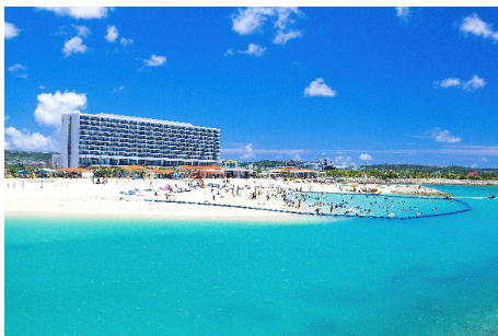
Appearance of Building
