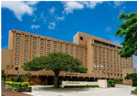
Appearance of Building
