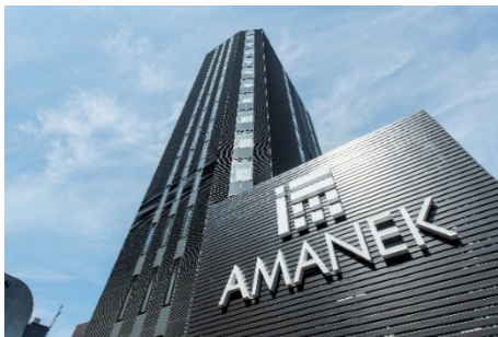
Appearance of Building
