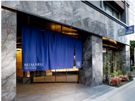
Appearance of Building
