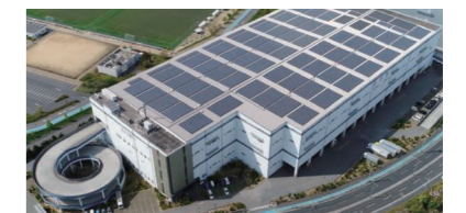
Solar panels at the Sakai Logistics Center
