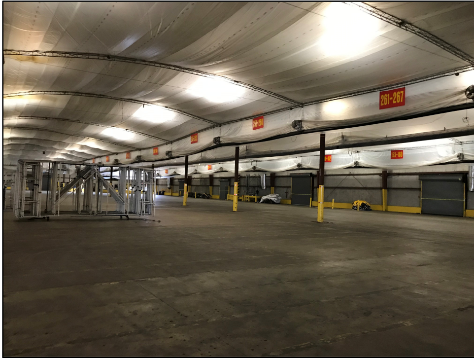
Photograph 1: View beneath empty shroud, Warehouse F.
