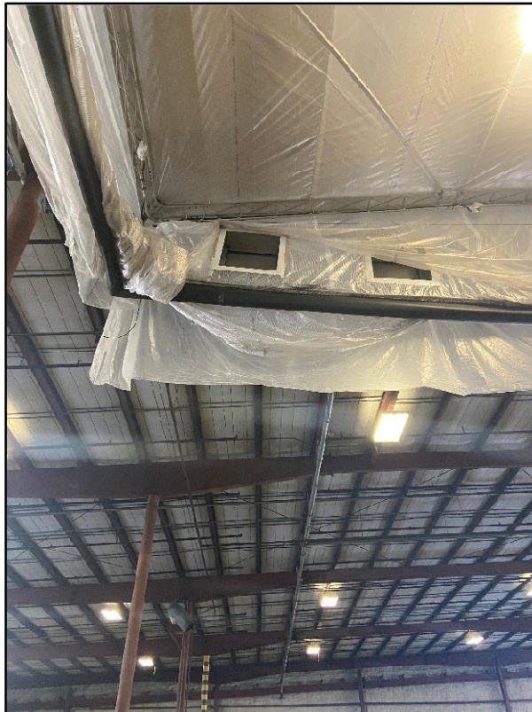
Photograph 4: Exhaust connection point on elevated shroud, Warehouse F.
