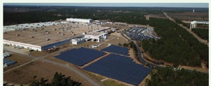
Aiken County, South Carolina passenger/light truck tire plant
