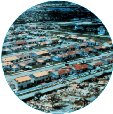
Building code assessment and mitigation
