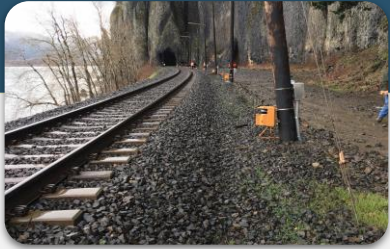
Rockfall Monitoring System
