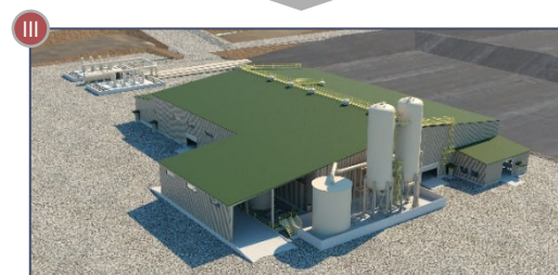
Merrill-Crowe process plant (capacity of 13,750 gpm 1 )
