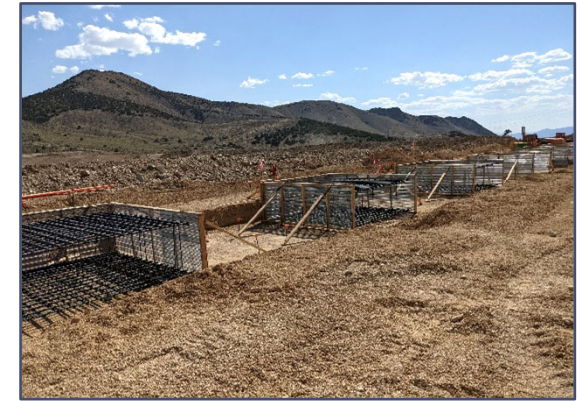
Formwork for Merrill-Crowe process plant foundation
