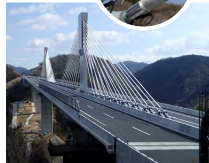
Shin-Meishin Expressway, Ikuno Bridge (NEXCO West Nippon)
