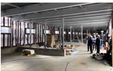
Building safety assessment
