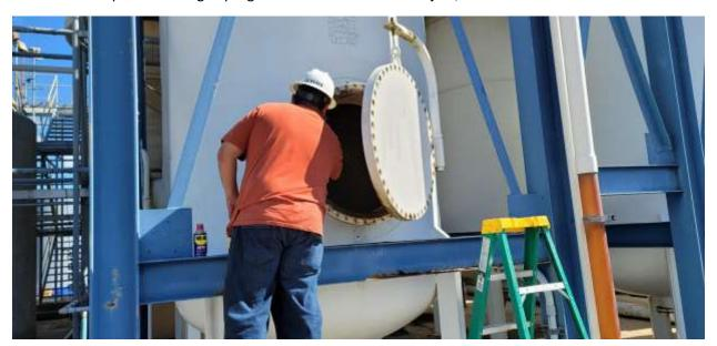
Above: An enCore Energy Corp. employee inspects one of the ion exchange resin elution vessels at the Rosita Central Processing Plant, South Texas.
