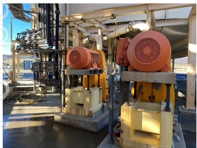
TAILINGS THICKENER PUMPS & MOTORS
