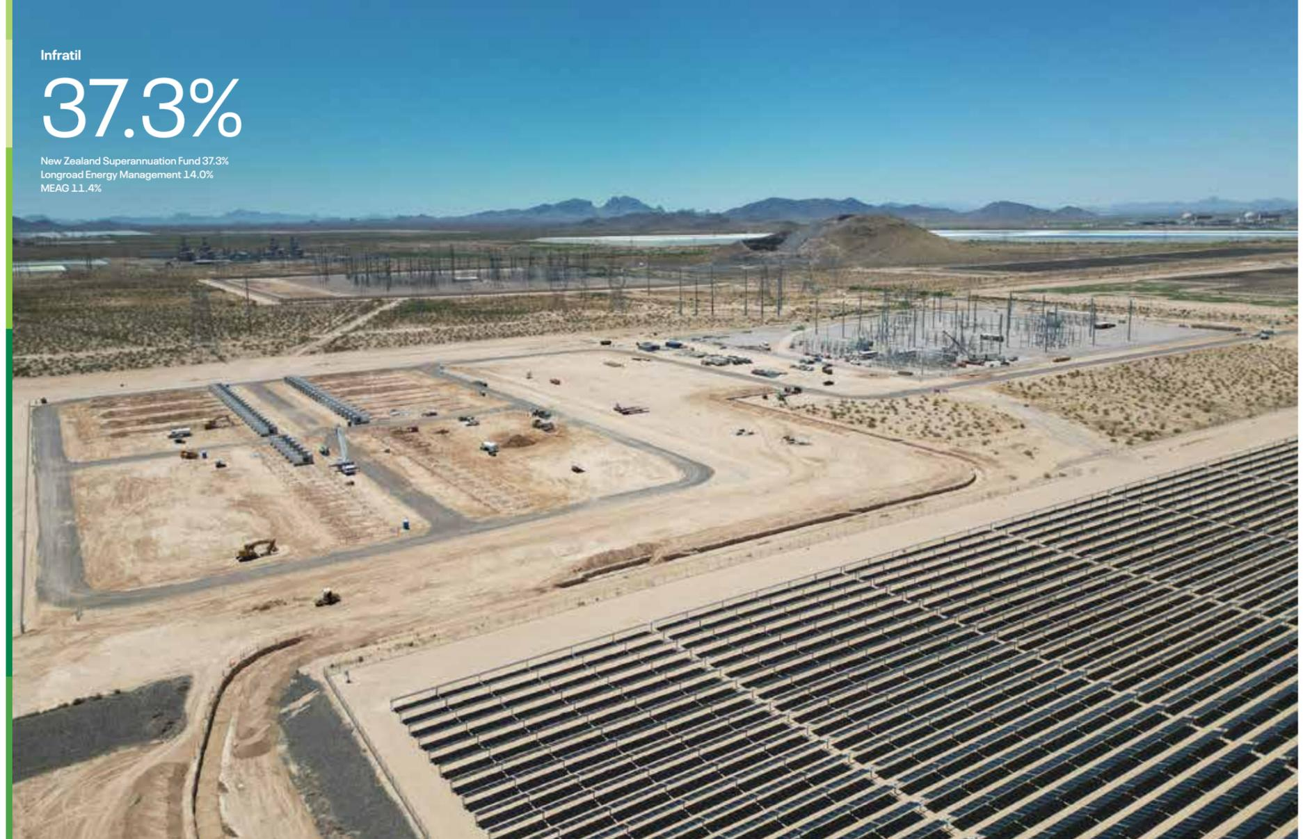
The switchyard and battery installation at the Sun Streams 4 solar farm, Arizona
