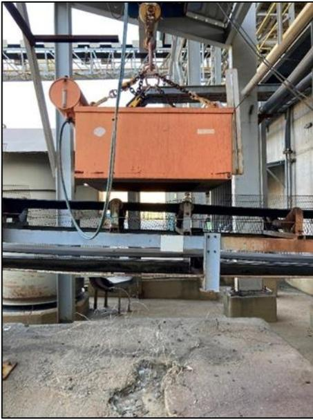
Figure 17-12 Magnetic Separator
