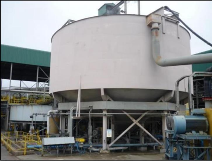
**Figure 17-29 Tailing thickener (Golder)**
