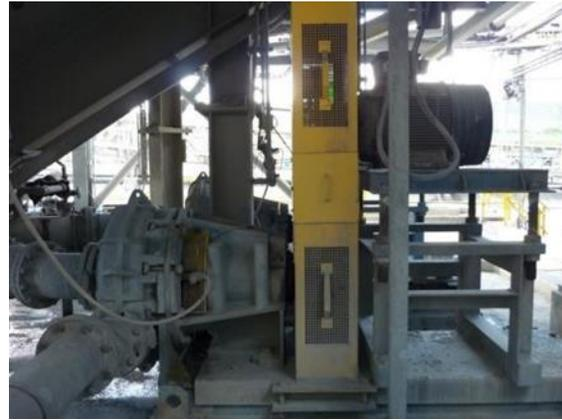
**Figure 17-31 Centrifugal pumps (Golder)**
