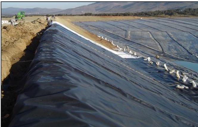
**Figure 18-4 HDPE liner on slope secured by anchor trenches**
