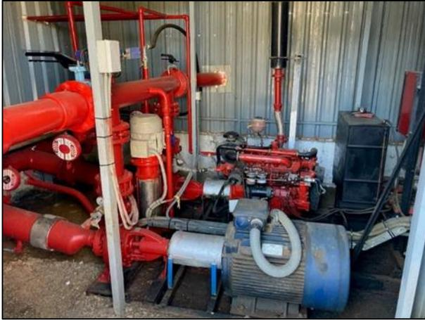
**Figure 17-35 Firewater pumping system (Lain photo)**
