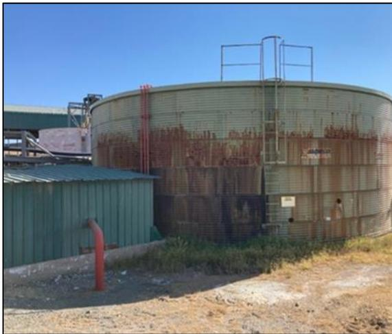
**Figure 17-34 Process water holding tank**
