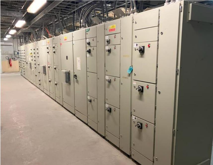
**Figure 18-3 Process plant ACC cabinets**
