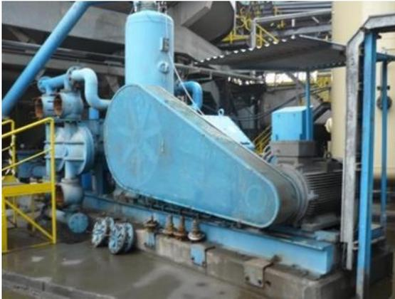
**Figure 17-30 Piston diaphragm pump (Golder)**
