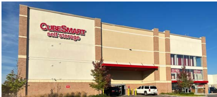
Industrial/Self-Storage 7% Tonelle Commons
