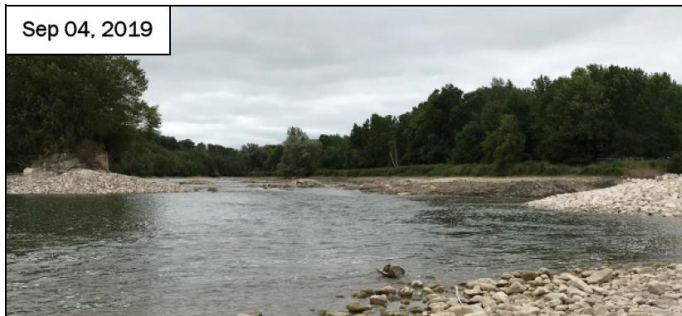
Figure 49 - Truax Dam, Walkerton, Ontario. The original wooden dam was built in 1852 and later replaced by the concrete structure shown above in 1919. The dam posed a significant barrier to fish passage for more than a century before it was removed in the summer of 2019 over the course of 3 weeks.
