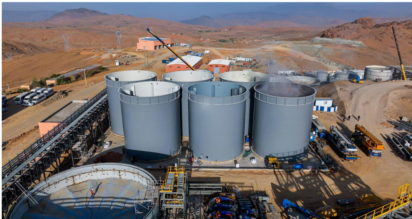
Figure 3 - Completion of the New Cyanidation Tanks at Zgounder
