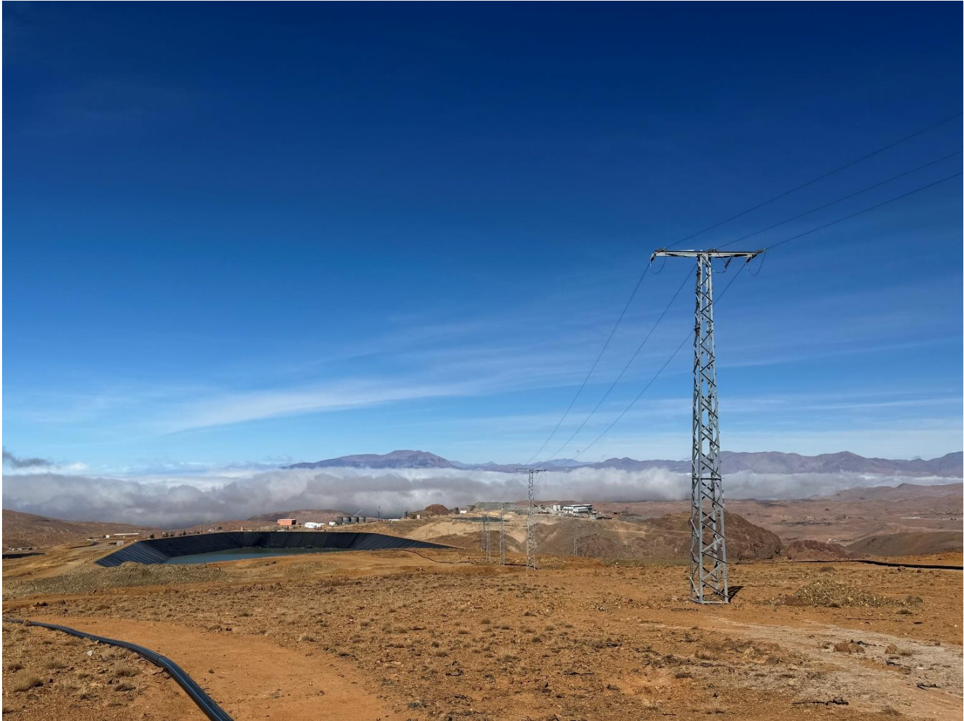
Figure 4 - Advancement of the Power Line Infrastructure
